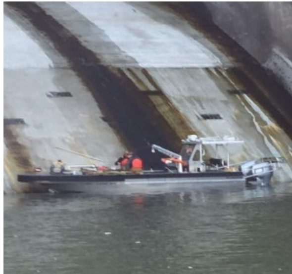
Figure 22. Work skiff providing access to the OGEE.
