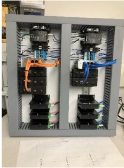
Figure 23. Upgraded communications panel ready for installation at PRO
