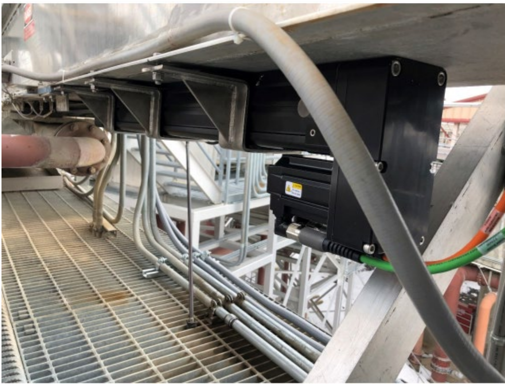
Figure 16. New electric cylinder at LMJ B-side gate
